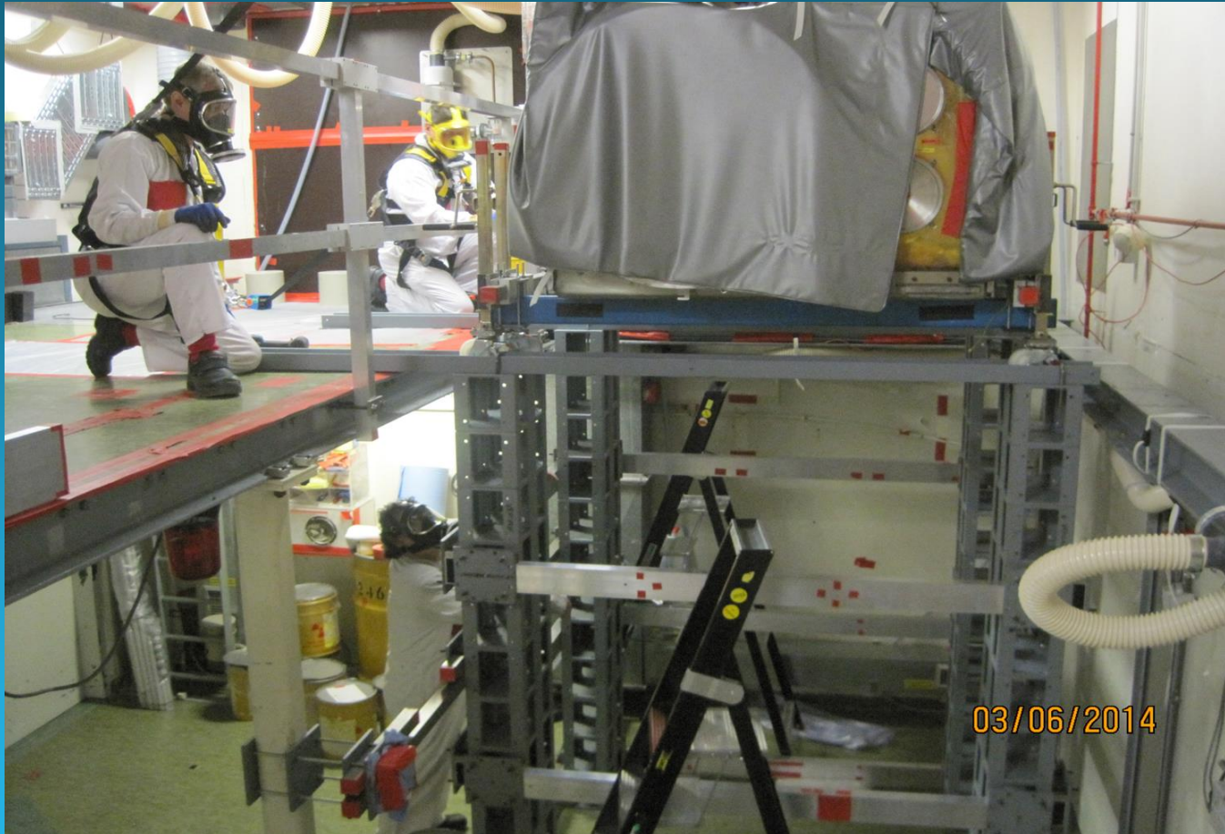
Moving a glovebox from a platform to the floor for decommissioning
