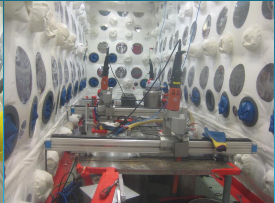
Automated cutting of 30 mm thick SS GB bottomplate
